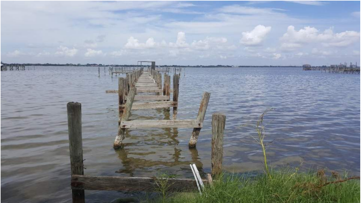
Picture 4: Existing marina/residential dock
