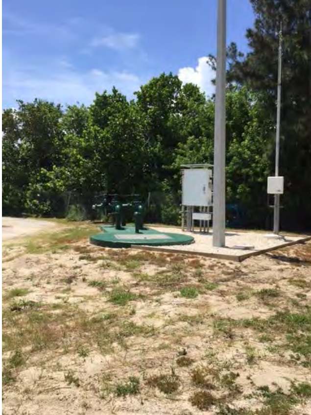
Photo 9. County lift station in the SE area.
