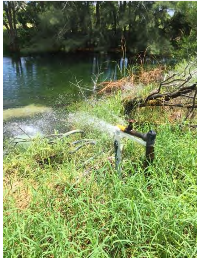
Photo 20. Free flowing water from leaking pipe
