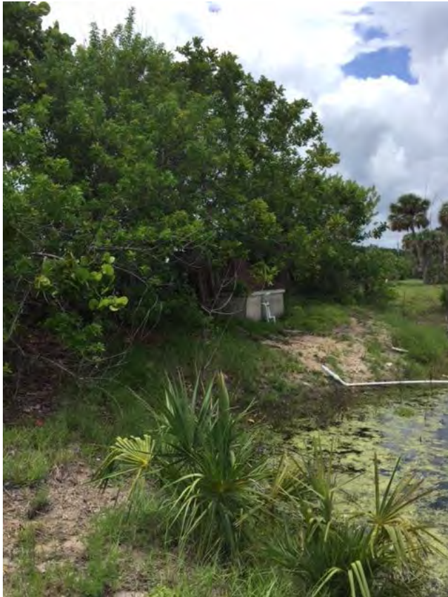
Photo 7. Small pump house.
