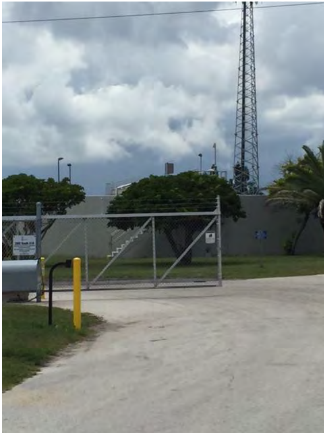
Photo 23. South Beaches WW Treatment Plant
