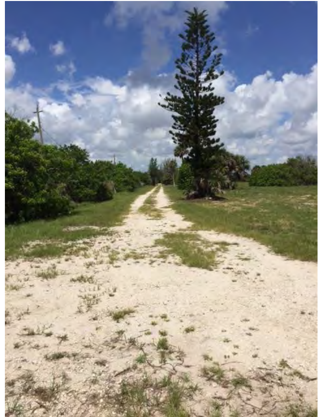
Photo 16. Road in south that runs east/west.
